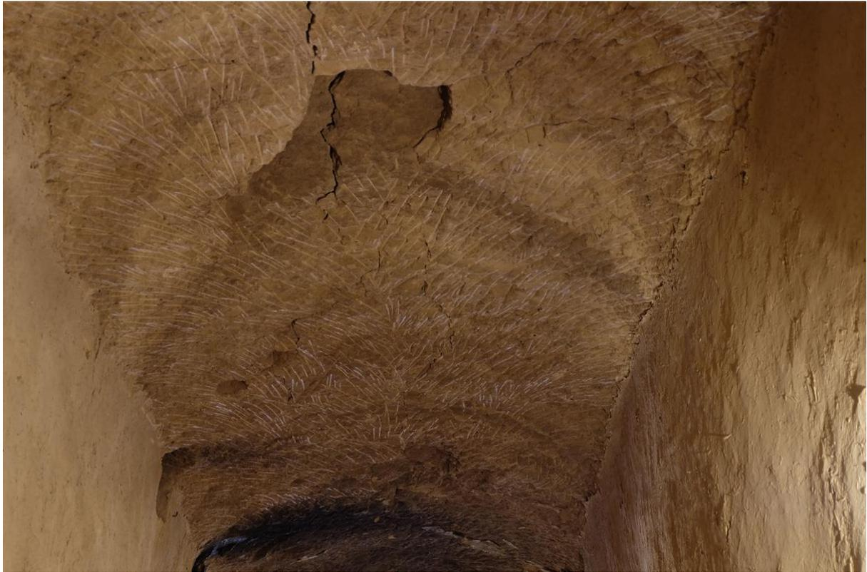
Figure. 8 Scratch markings made by digging axes on the roof of the corridor
