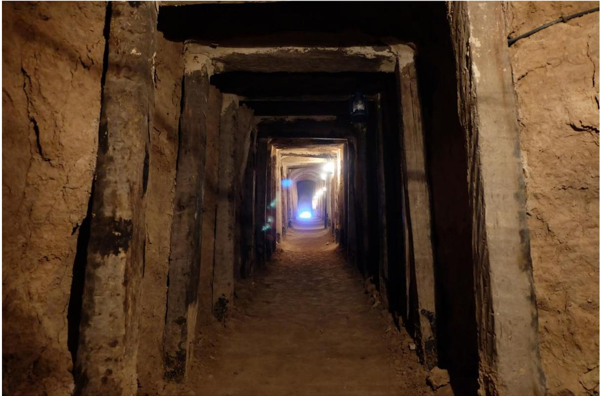
Figure. 10 Wooden frames added to reinforce the damaged roof of the corridor
